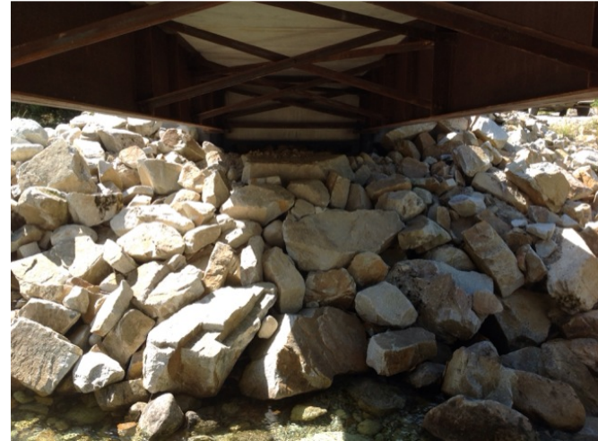
Left Bank Abutment when facing downstream
