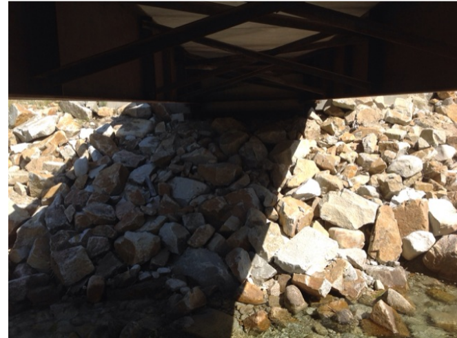
Right Bank Abutment when facing downstream
